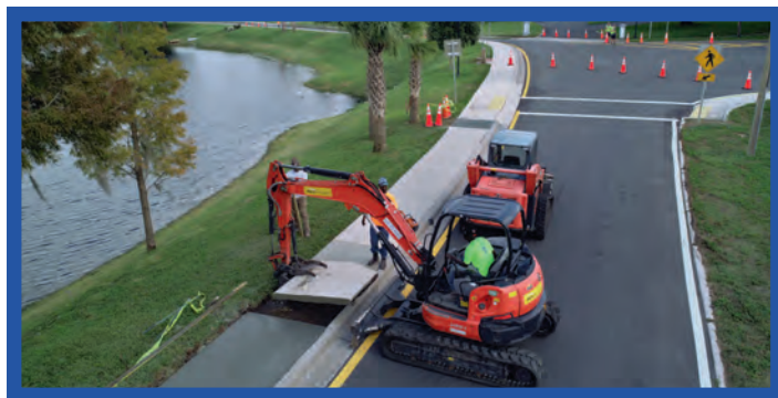
Top-left: Removal of a section of sidewalk for replacement
