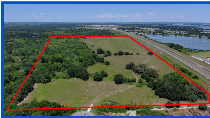
Hickory Road Sprayfield.
