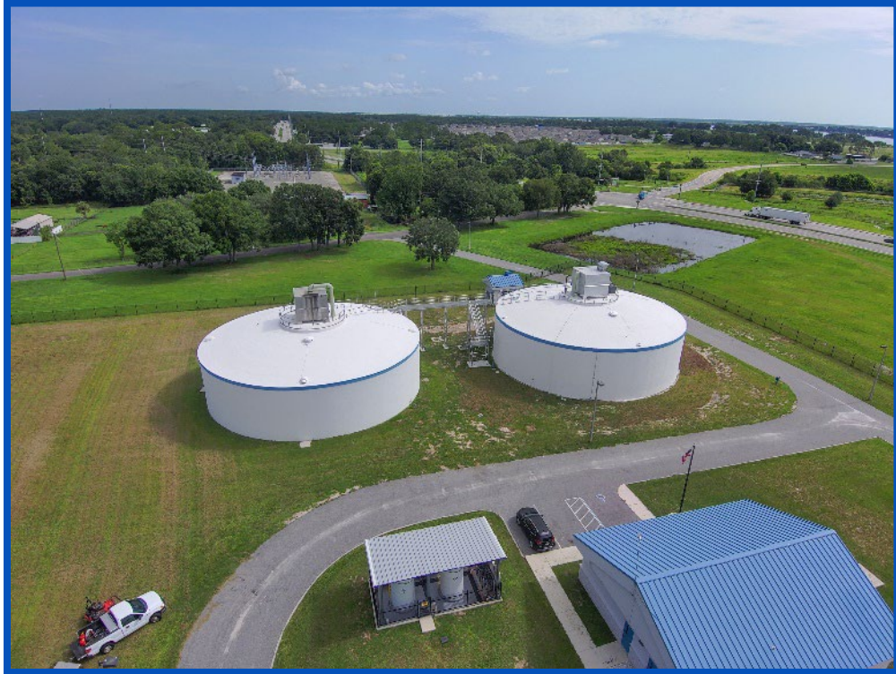
Aerial View of the Berkley Water Treatment Plant Expansion.
