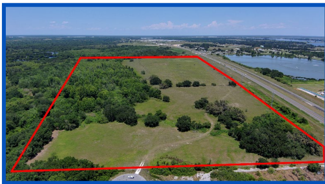
Hickory Road Sprayfield.
