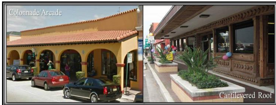
Figure 15.3-15. Colonnade, Arcade, Cantilevered Roof
