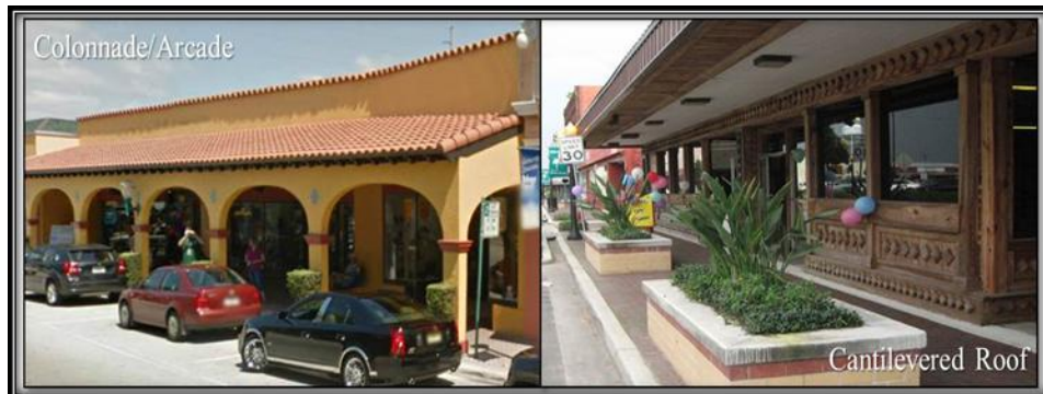
Figure 15.3-15. Colonnade, Arcade, Cantilevered Roof
